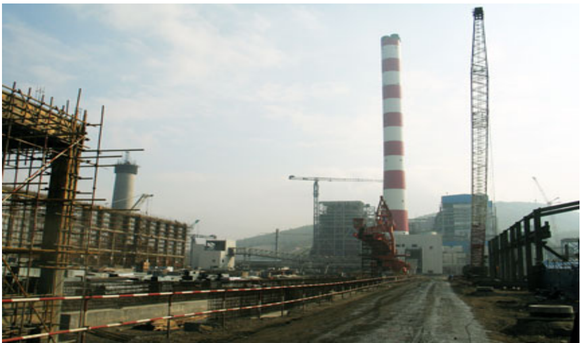
Construction site of a coal-fired power plant
