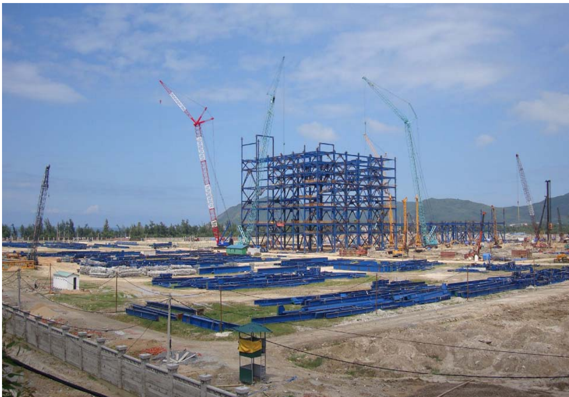
Vung Ang 1 Power Plant Construction Site as April/2010
